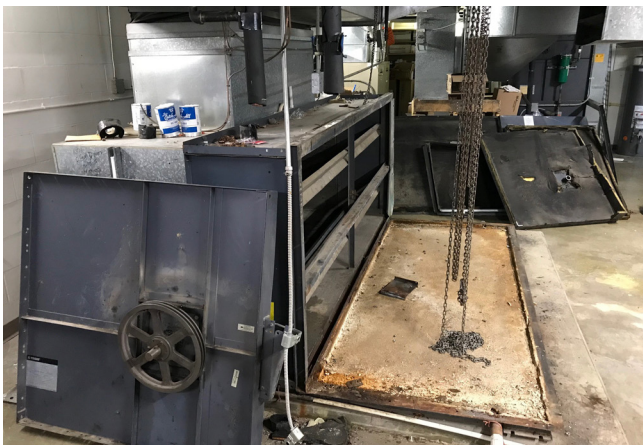
Old air handling system
