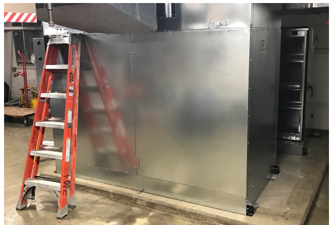
New air handling system
