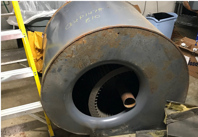
Old blower motor
